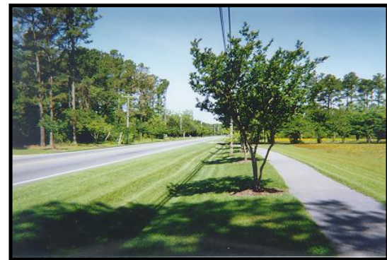
Shared-use path parallel to a roadway photo by Phil Hinton
